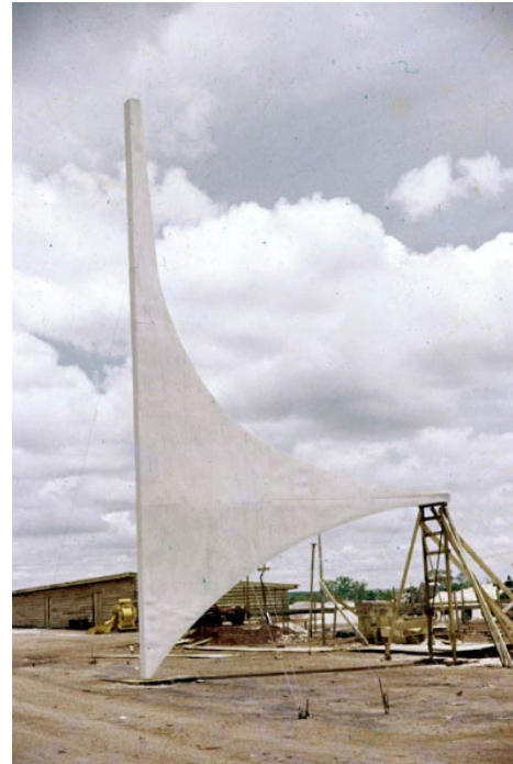
Mário Fontenelle, Prototype of Oscar Niemeyer's column at Brasília's construction site , ca. 1958. Photograph, 3 7/8 x 5 7/8 in. Courtesy Arquivo Público do Distrito Federal, Brasília. From the 2026 grant to Ciro Miguel for the publication Brasília in 35mm: The New Capital through the Lens of Photojournalism, 1956–60
